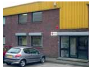
Installations Office (North) Salford, Manchester
